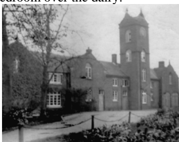
Bellaport Hall Farm with the tower - later demolished.
