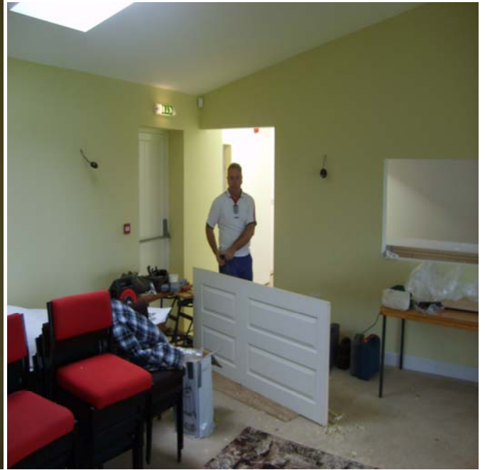
Ian Groom hanging 1 of the 9 interior doors – Only another 4 to go !!
